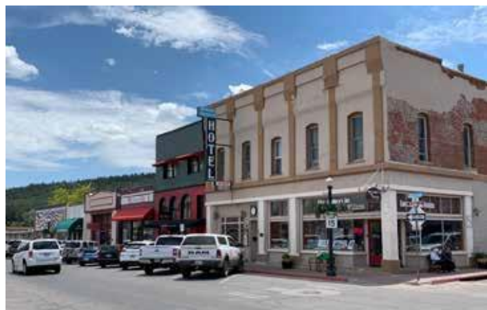
Figure 3: Typical Roof Parapets
