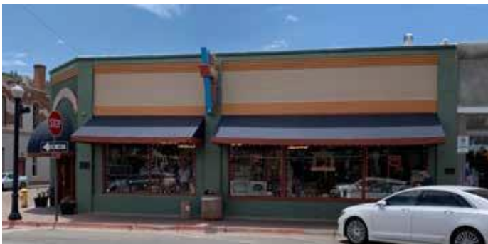
Figure 35: Multiple Awnings over Doorway and Storefront
