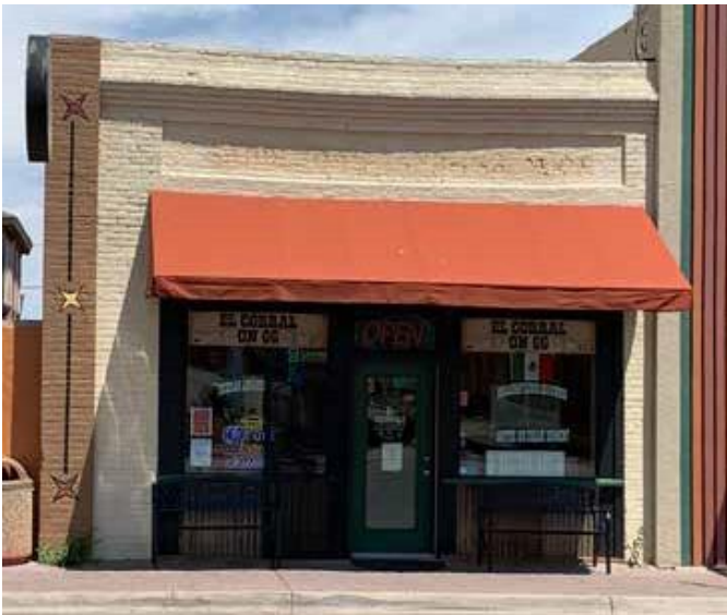
Figure 33: Awning over Storefront
