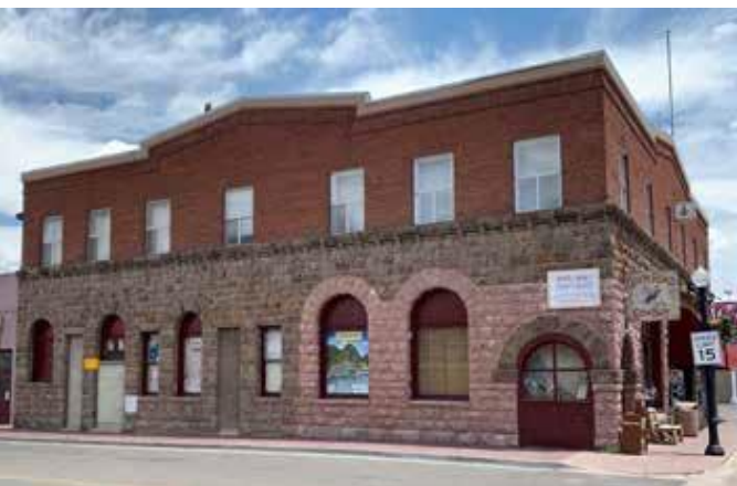
Figure 17: Second Floor Vertical Windows
