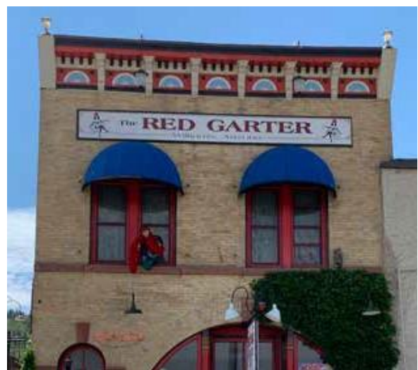
Figure 36: Second Floor Awnings
