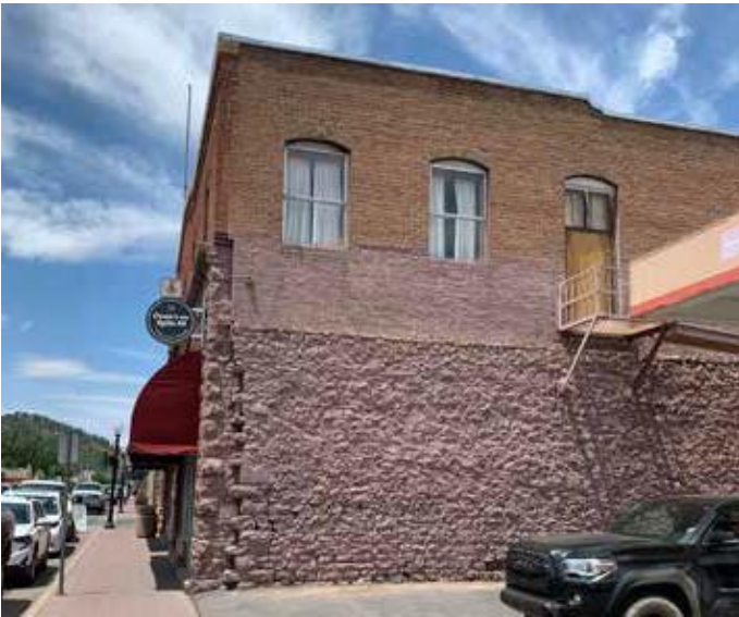
Figure 25: Mixed Masonry Types (brick and stone)
