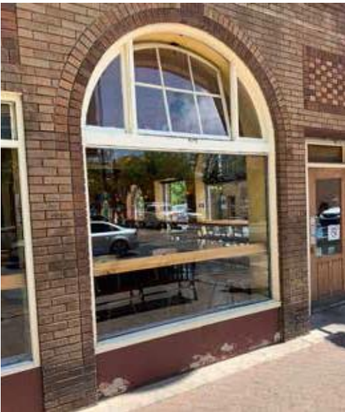
Figure 15: Preservation of Original Wood Window
